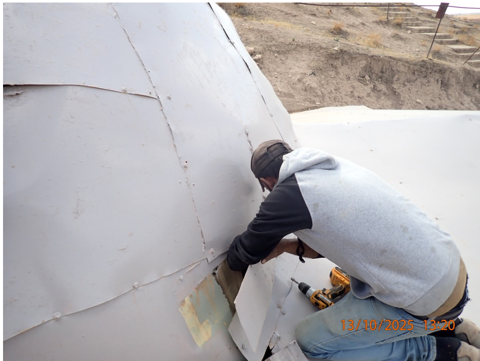
Fig. 10: The re-installation of a missing bolt on the Abi dome
