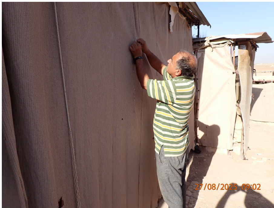
Fig. 1: Stitching of the Burlap in the Palace Area
