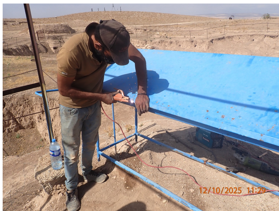
Fig. 4: welding of minor cracks in the temple panorama
