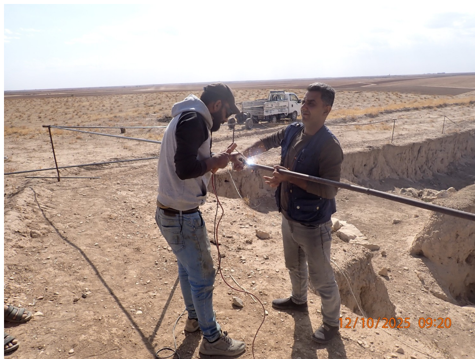
Figure 3: welding of the rods
