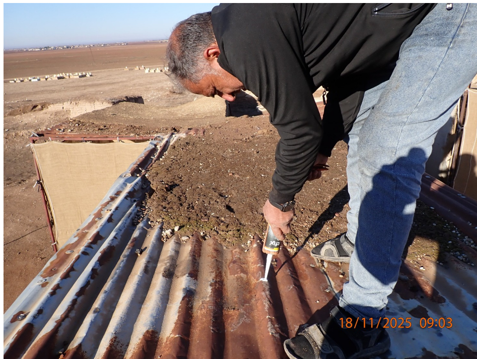
Fig. 14: Sealing gaps and existing holes in sheet metal (tutiya) with silicone
