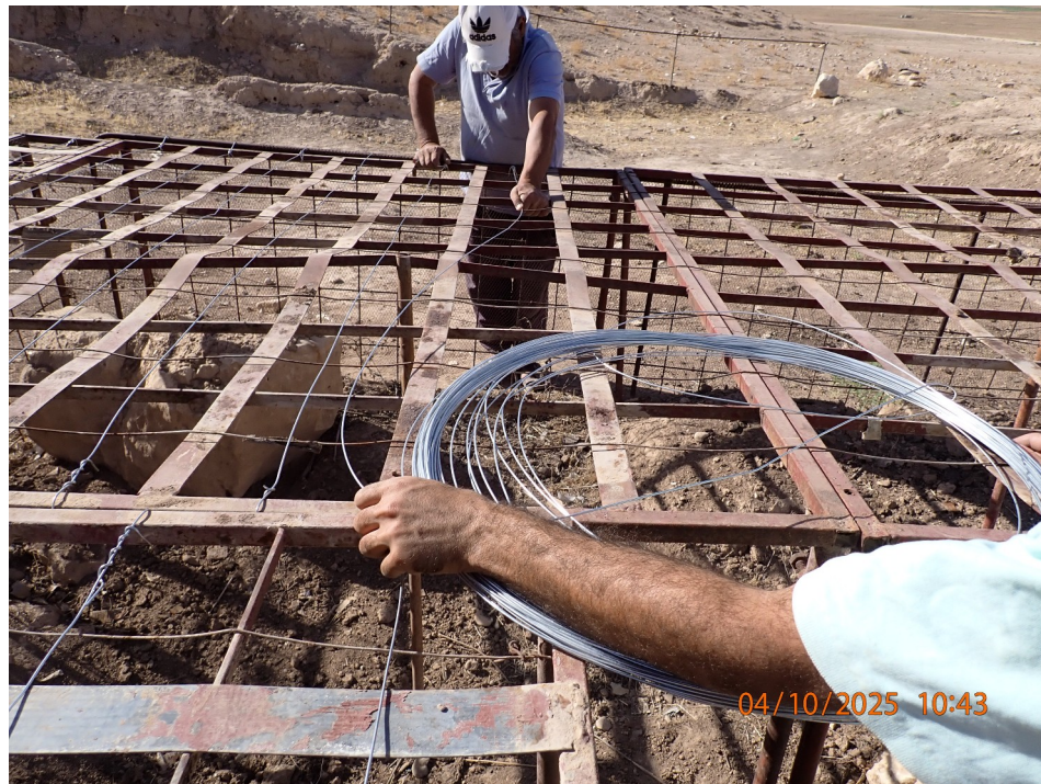
Fig. 12: Metal wires installation
