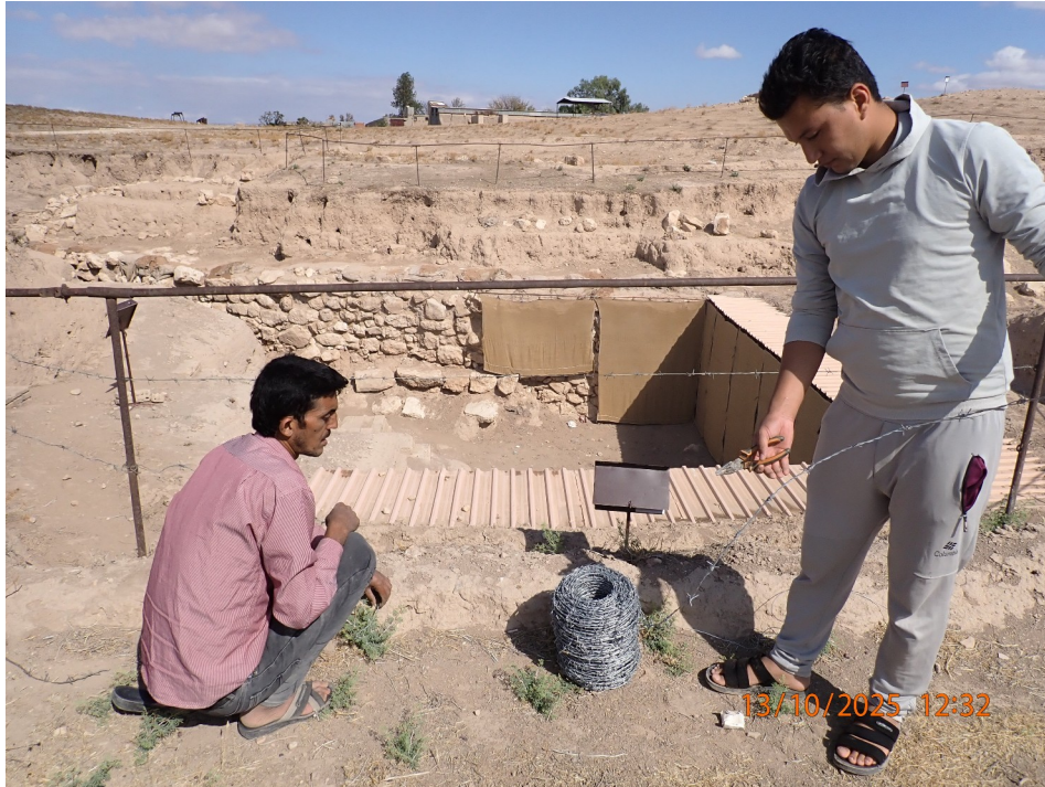
Fig. 9: The reinstalling of the new protective barbed wire
