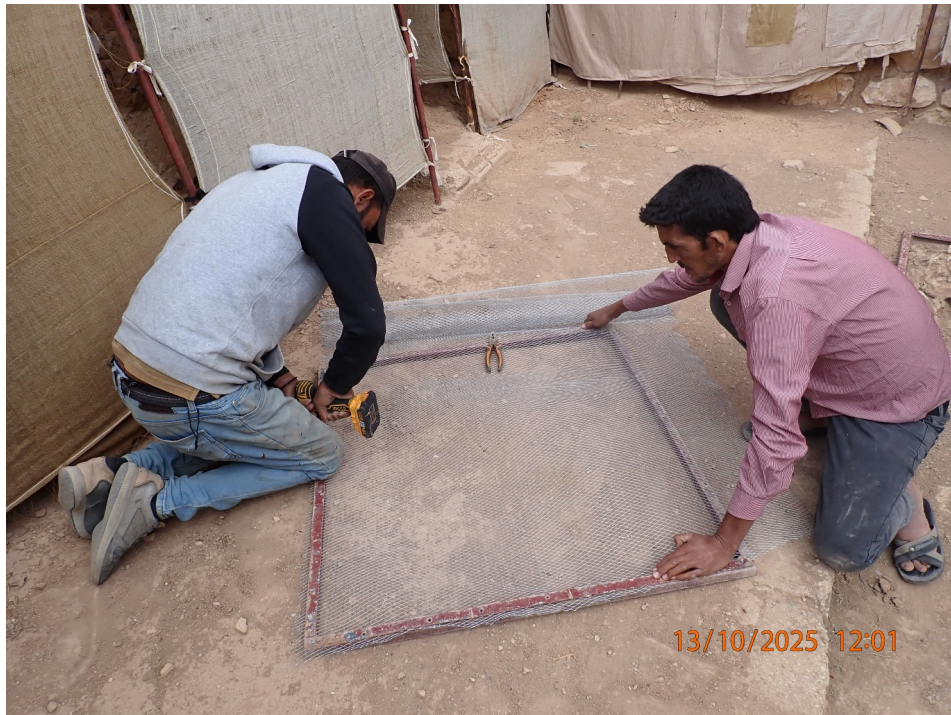
Fig. 7: The installation of the new mesh on the drainage frames
